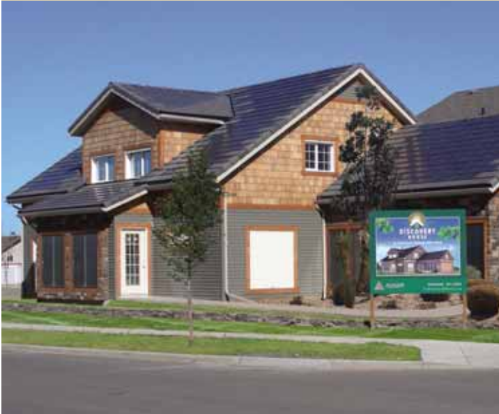
Photo Credit: Avalon Master Builder
